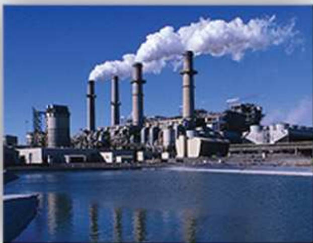
Fossil fuel power plant
